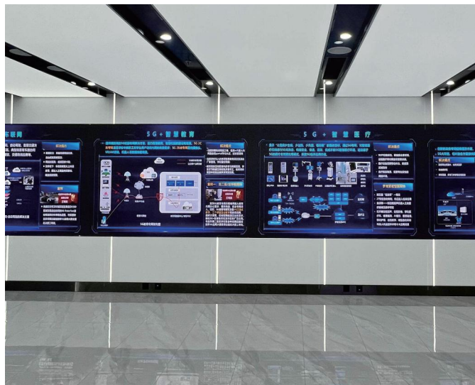
Command and Control Centers
