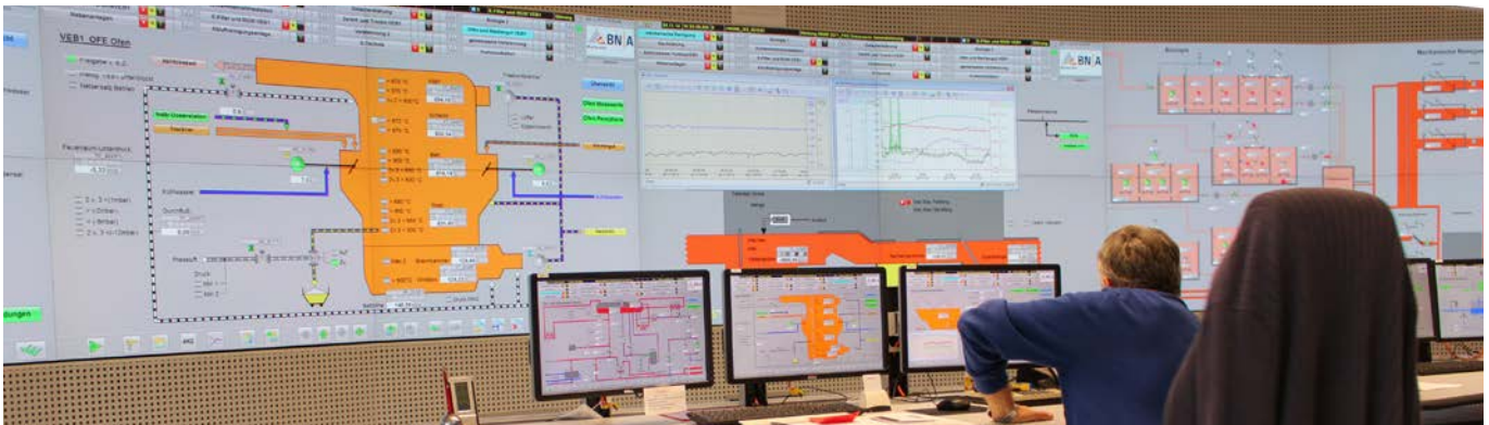
Water Purification — Karlsruhe, Germany Rear Projection Video Wall (9x2 of 60" Full-HD)
