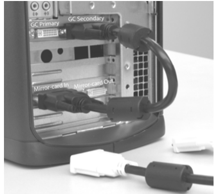
Short DVI cable installed
